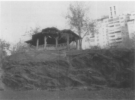
Figure 35-37: Central Park has developed an in-house historic preservation crew to undertake small projects. A specialized crew has been trained to specifically repair and rebuild rustic furnishings. As illustrated, the restoration of the Dene rustic shelter was achieved by constructing it in the Ramble compound, moving in-place opposite 67th street and completed. (courtesy Central Park Conservancy)
